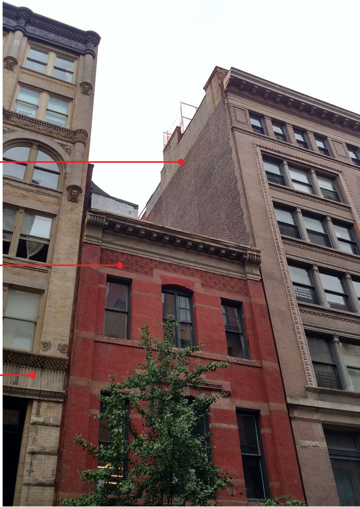
Existing Mechanical bulkhead @ 101 Wooster
