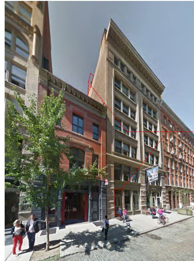
2. Exterior view from Wooster St (looking N)
