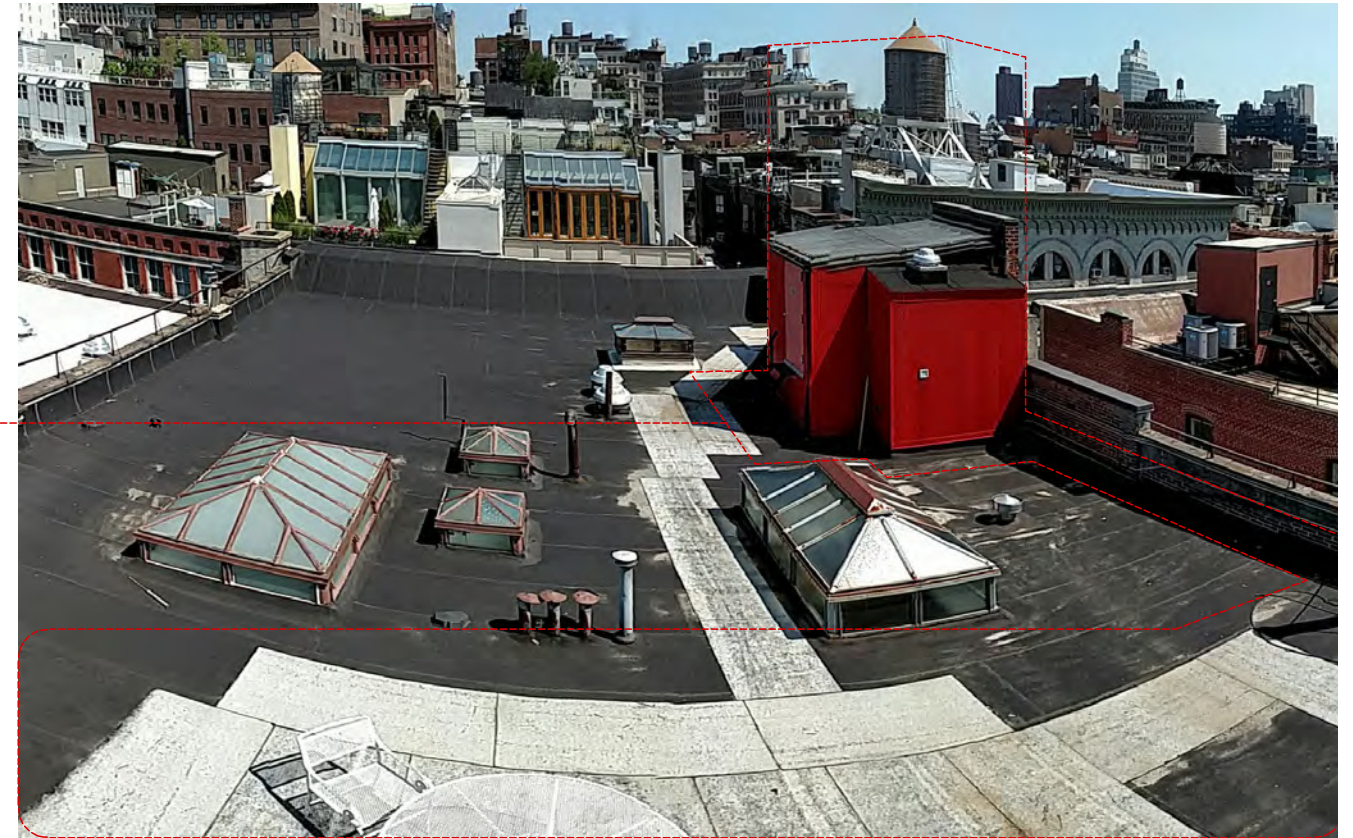
3. View of bulkhead from roof
