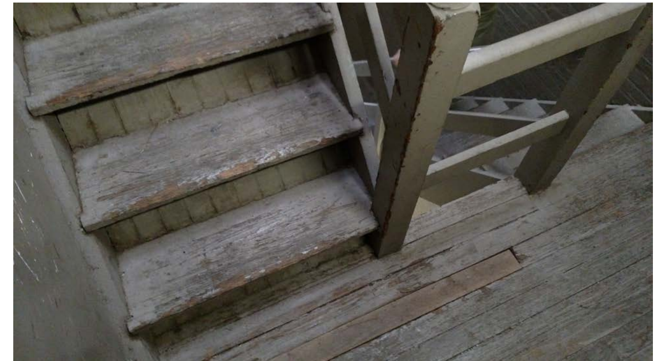
04 existing stair condition nts
